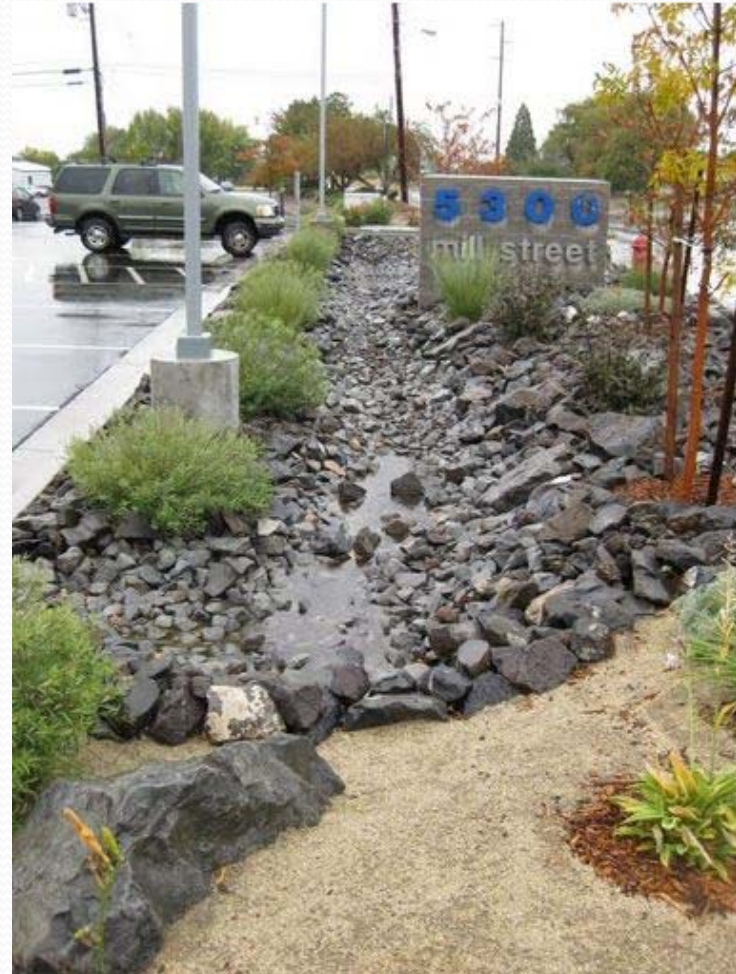
United Construction parking lot swale
