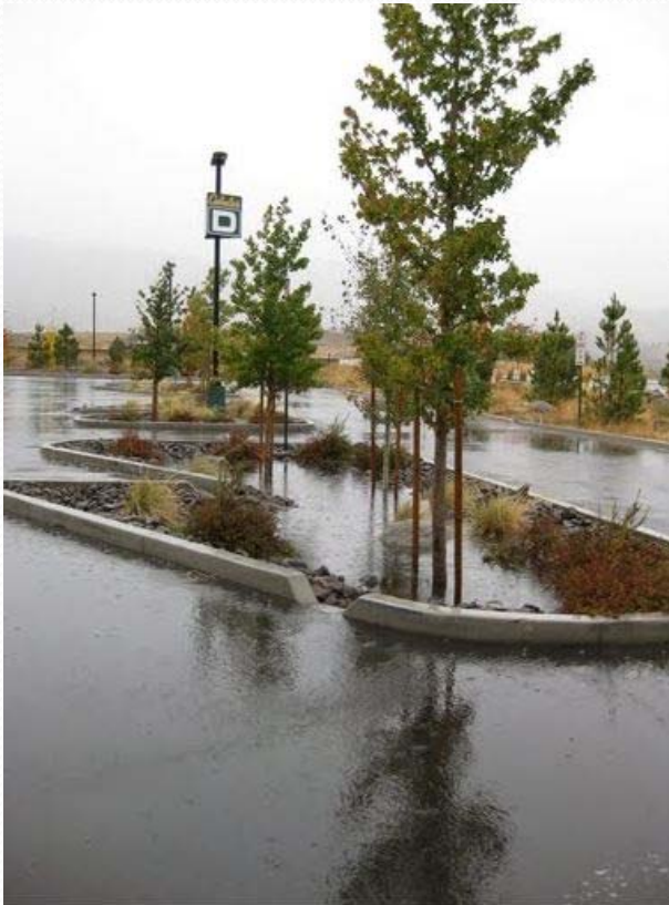
Cabela's curb cuts and parking lot islands
