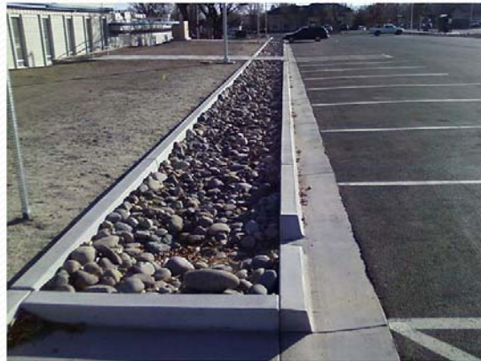
Carson City Community Center infiltration feature with curb cut
