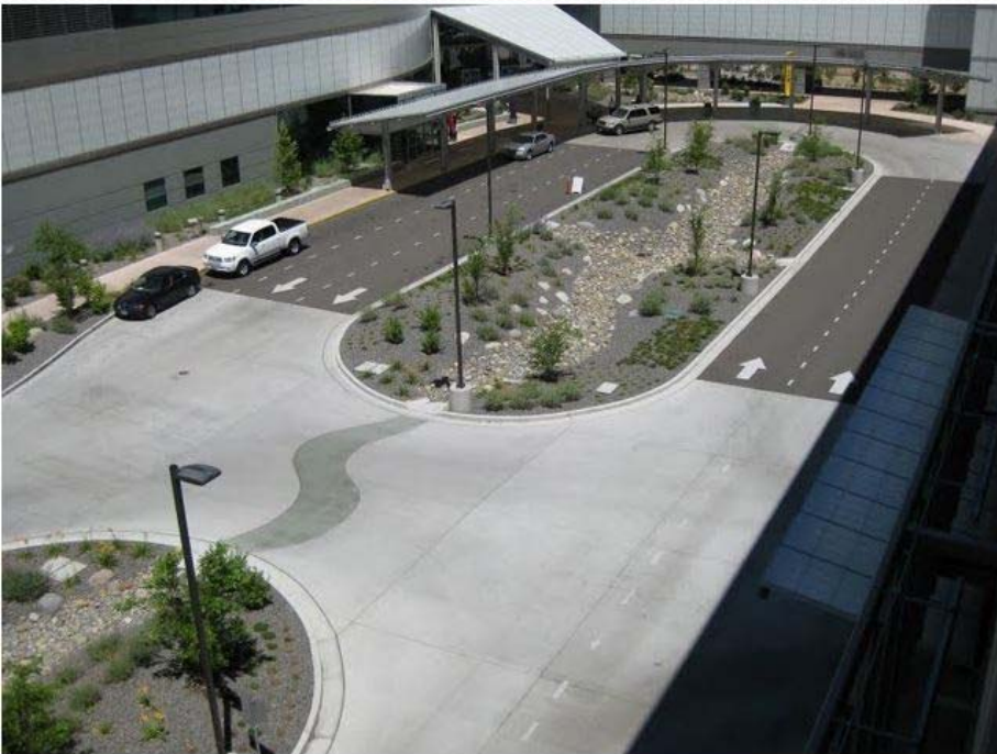
Renown rock-lined swale
