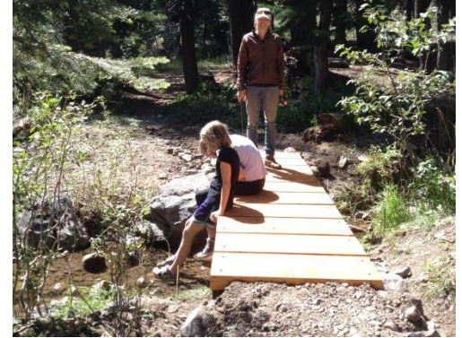
Trout Habitat Enhancement Bear Valley Bridge built to prevent trail erosion
