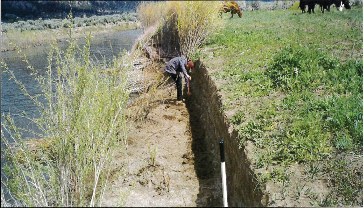
Crew installing a vertical willow mattress at the Kermin track
