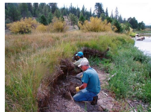
Hope Valley Willow Staking Hope Valley 375 willow stakes planted 300 feet of stream bank stabilized
