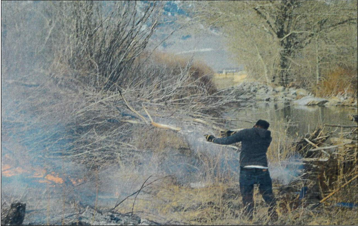
Burning flood debris and slash materials near Lutheran Bridge.
