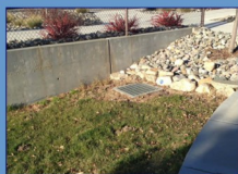
By stabilizing the area with vegetation, this BMP prevents erosion
