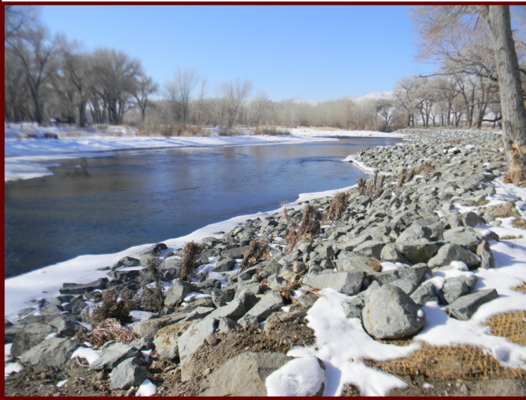
The stabilized stream bank after restoration work was completed on the Middle Carson River in Dayton.
