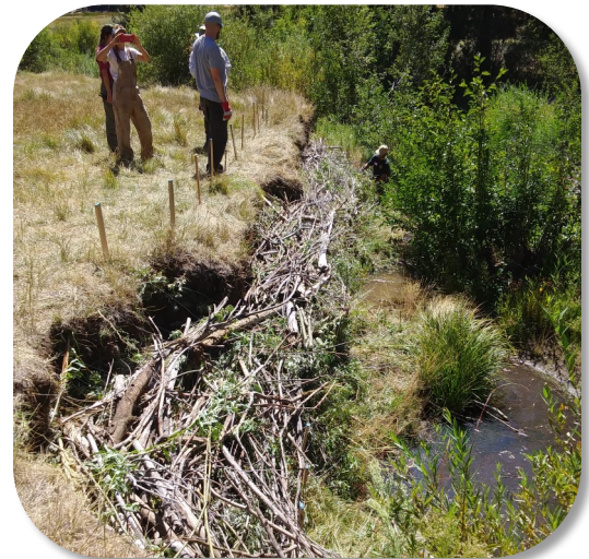
Stream bank after stabilization with brush boxes. Photo by Justin Bedocs
