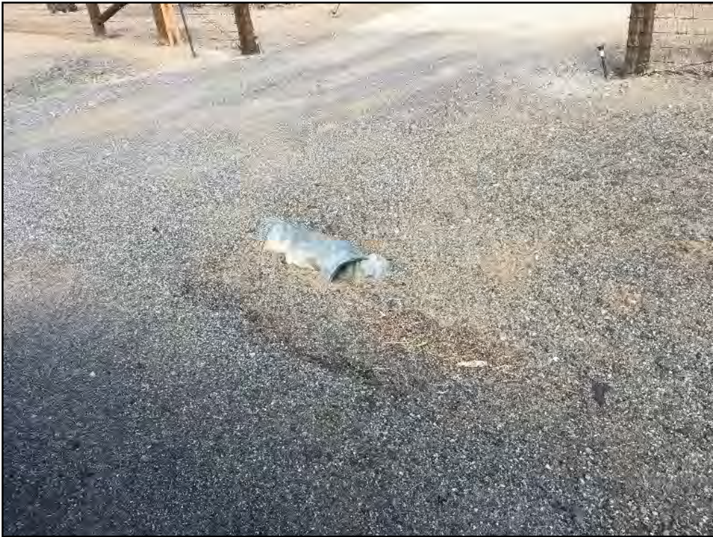
Figure 5-6. Examples of typical driveway culverts in study area (note sediment clogging and available headwater depth).
