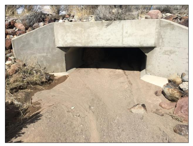
Figure 3-1. Example of sediment deposition at culvert
