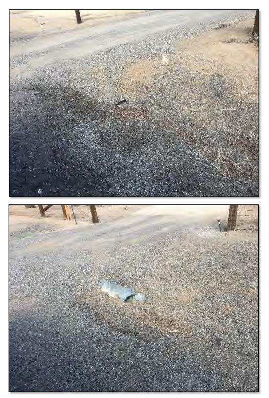
Figure 5-6. Examples of typical driveway culverts in study area (note sediment clogging and available headwater depth).
