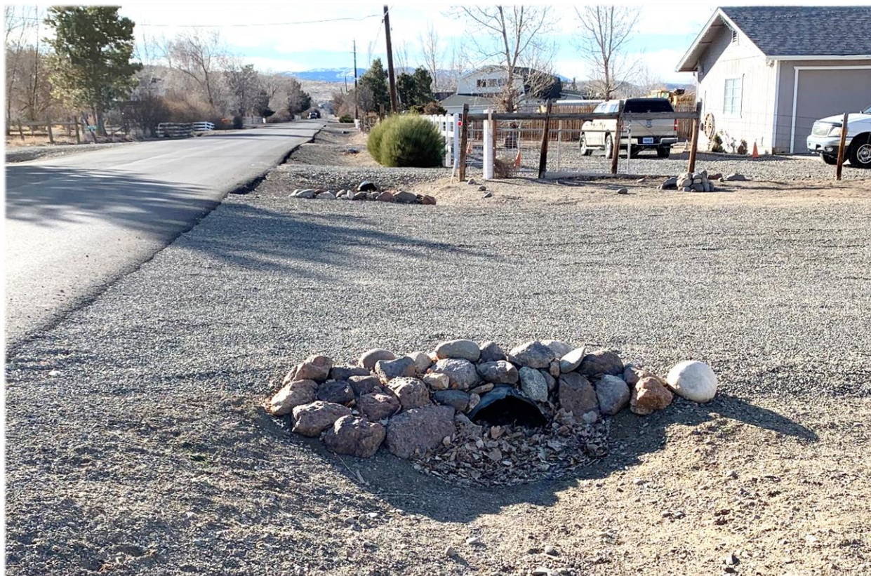
Figure 2-12. Typical driveway culverts
