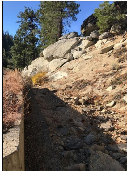
EXISTING UNDERSIZED SPILLWAY
