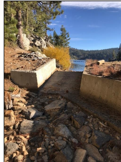
EXISTING UNDERSIZED SPILLWAY
