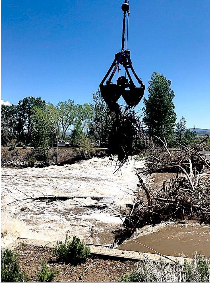
Logs and debris are lifted away from a logjam at the Virginia-Rocky Slough diversion on the East Fork of the Carson River by Connelly Crane. Tod Carlini/East Fork Fire Protection District
