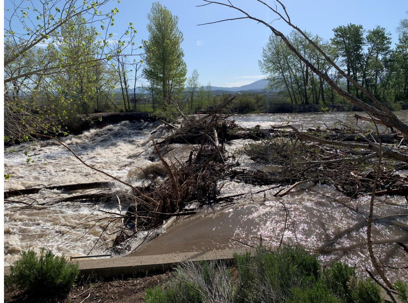
Irrigation Ditches overflowing from diversions in Carson River
