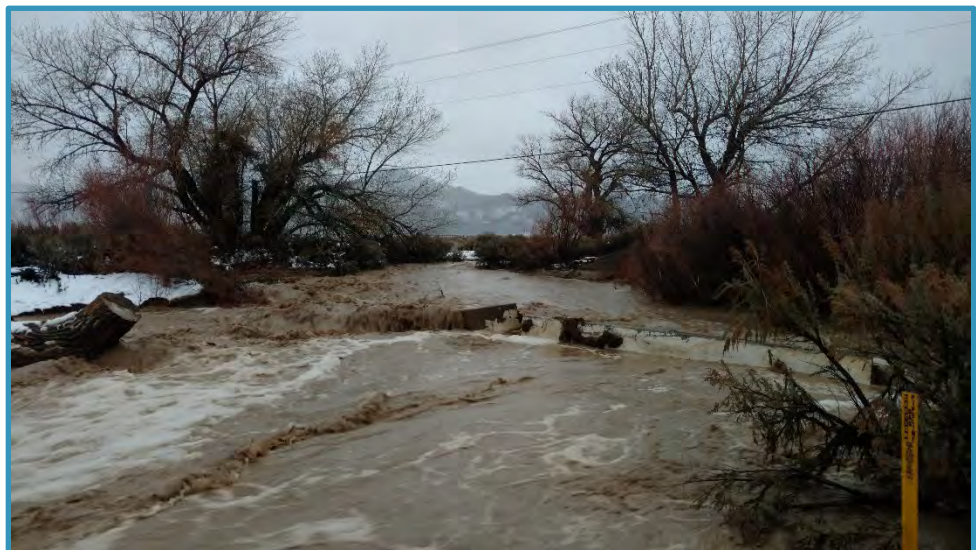
Figure 54: Diversion Structure in Dayton damaged by 2017 flood. Ed James
