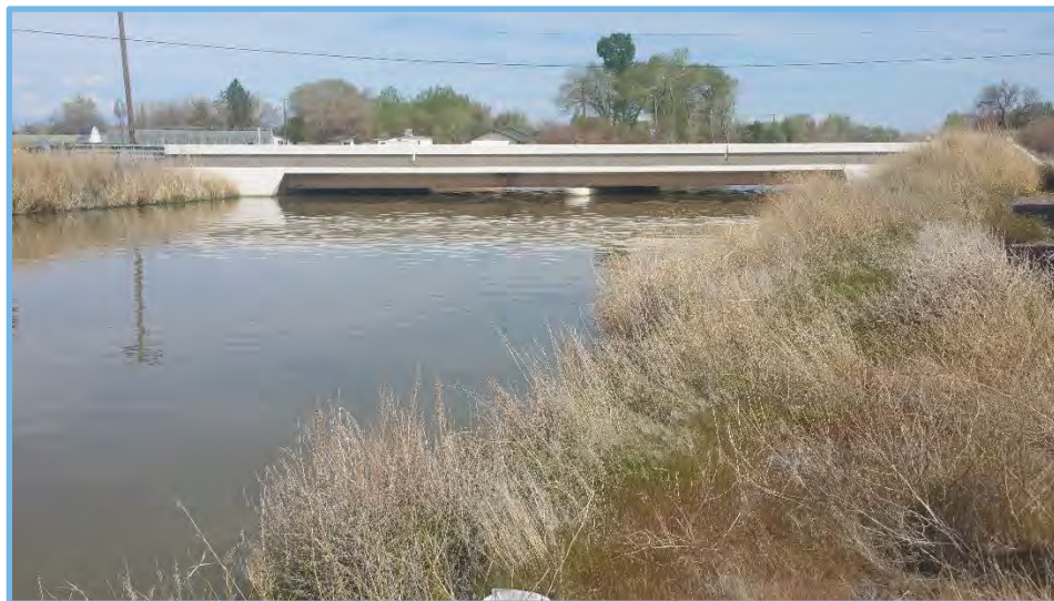
Figure 41: Bafford Bridge, Churchill County. Brenda Hunt 2017
